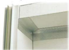
Top and underside view of ceiling support system detail showing 40 x 40 x 3mm L-shaped mild steel profiles screwed horizontal to the 50mm thick partition and ceiling panels with steel self-driving screws every 800mm or less
