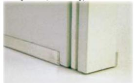
Floor detail showing 50 x 50 x 20 x 3 mm U-shaped mild steel profiles screwed horizontally to concrete floor with concrete anchors every 800 mm or less
