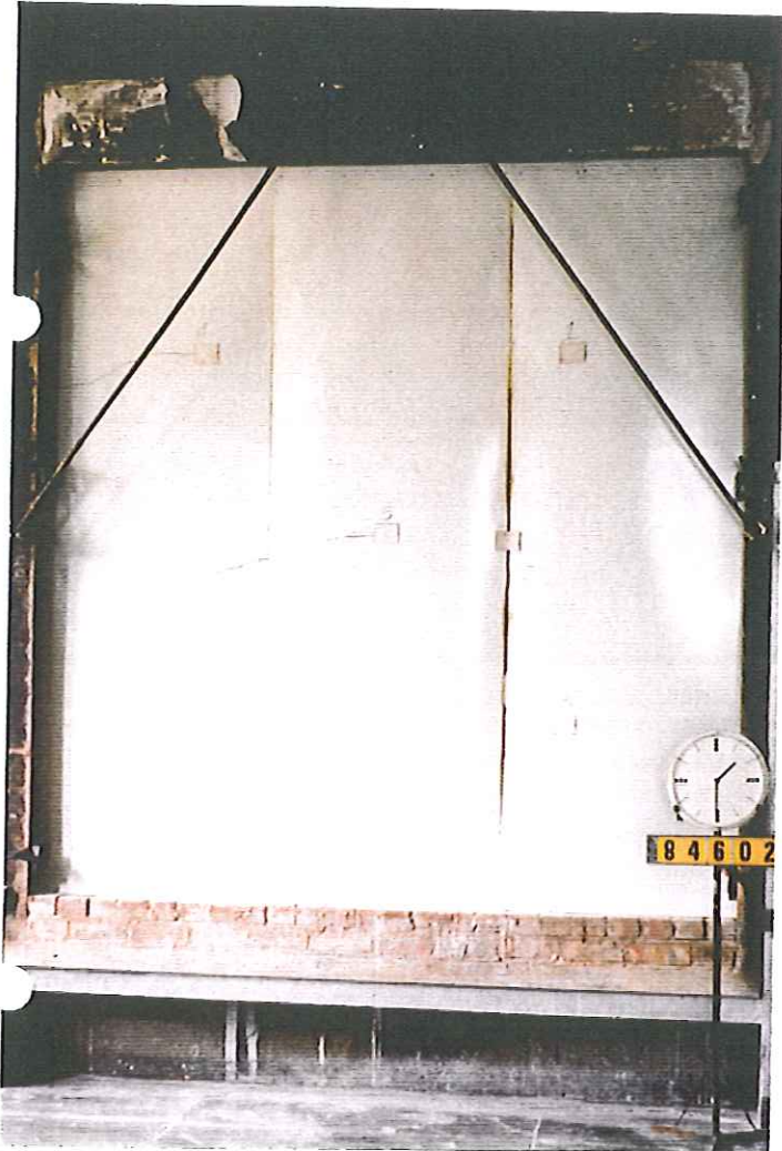
No 5 Panel at termination of test: 90 min
